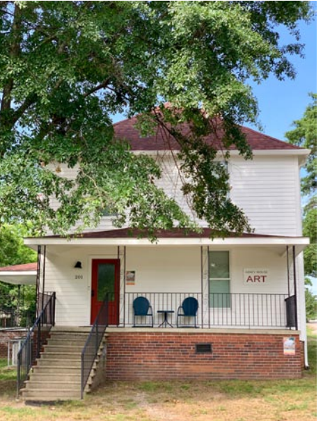
Photo of the Abney House
