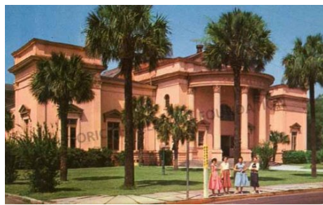
Thomson Auditorium built in 1899, as a convention space for the United Confederate Veterans reunion, later became the home of The Charleston Museum in 1907, which was located at 121 Rutledge Avenue. (Source: The Buildings of Charleston by Jonathan Poston.) The featured color photographic postcard was published by Colourpicture Publishers, ca. 1960s.
